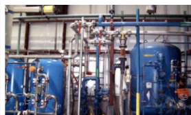
Piping Fabrication All Types of Piping Fabrication & Installation
